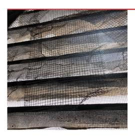
**ISSUE 7**View of one of the four gable vent interior screens showing its cobbled together.
