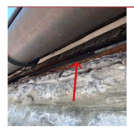
Close up of some prior sealing work along roof edge. Here backing material of 1/4" welded wire is present
