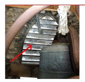
One of the four gable vent interiors in the bell tower. Interior screening is present, but not all in good repair and we recommend exterior screening for best protection.
