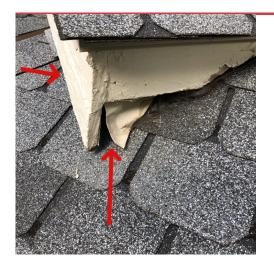
This eave end needs bent back into place and underside has exposed wood and small gap; recommend cladding with flashing and sealing.
