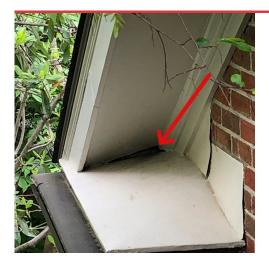
Primary animal entry point at construction gap in this gable end inside corner (flying squirrels strongly suspected)
