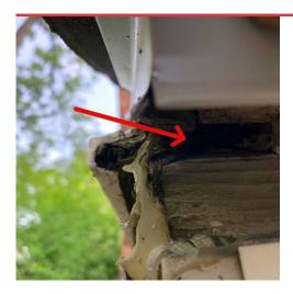
ISSUE 31 Close up of Issue 30 showing small gap to seal at this roof corner.
