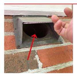
Higher bathroom exhaust with flapper held out has no screen and so is animal entry vulnerable.
