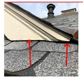
**ISSUE 20** Construction gap at this eave end needs sealed.
