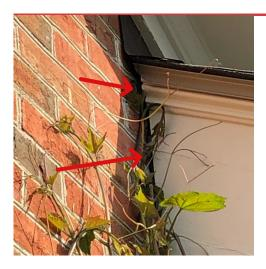
**ISSUE 28** Construction gap at end of this eave "eyebrow" to seal.
