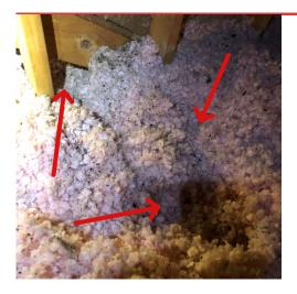
Trails observed in attic insulation consistent with size of flying squirrels.
