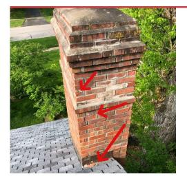
**ISSUE 27** Brick spalling observed on chimney.
