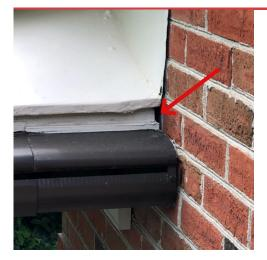
**ISSUE 29** Small construction gap to seal at this eave "eyebrow."
