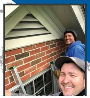
Following animal removal, we exclude animal intrusion with an exterior installation of steel welded wire, trimmed with custom-fabricated aluminum flashing. From mice to raccoons, all animal intrusion is denied, AND with style!
