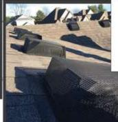
Squirrels chew through a variety of static box roof vent styles as seen to left, and loose installations or build welds can leave these vents vulnerable to mice, bats, raccoons and everything in between.
