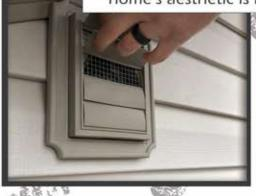
Bird nesting in dryer vents causes inefficient clothes drying as moisture can't escape, damaged heating elements in your dryer, and a risk of house fire.
