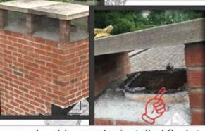
Screens should never be installed flush to a flue top like this, code was violated and a raccoon still defeated. We'll properly install stainless steel chimney spark arrestor material at the masonry openings for a safe, proper, and long-term solution.
