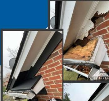
Squirrels and sawzalls can both make big holes on your home. Following animal removal we provide an exclusion repair above and beyond typical construction and steel clad the vulnerable areas. Impenetrable to future wildlife instrusion and once painted uncompromising aesthetics!
