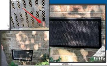
This plastic foundation vent poses no obstacle to mice. We install premium XclusionPro® Foundation Vent Guards from AAC Distributing to both protect and maintain access to the vent slider.
