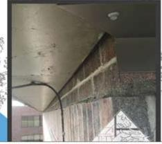
Common construction gaps on many residential and commercial buildings are sufficiently large to allow bat, mice, snake, and other small animal entry with little to no effort. Custom flashing installations are one method we use to close gaps with aesthetics in mind.
