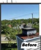
Galvanized steel chase covers on many modern gas flue systems rust and stain. Custom stainless steel chase covers are the solution we provide.
