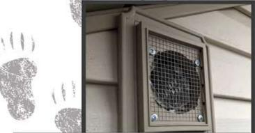
We stop bird entry at bathroom exhaust vents with inconspicuously installed steel welded wire rather than unattractive cages.
